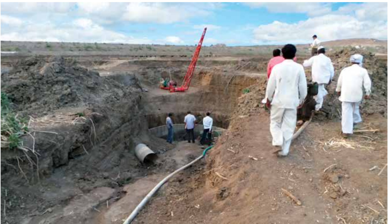
A well was dug in the dried up percolation tank to provide water to Mirkhala village. We provided technical support by installing PVC pipes.
