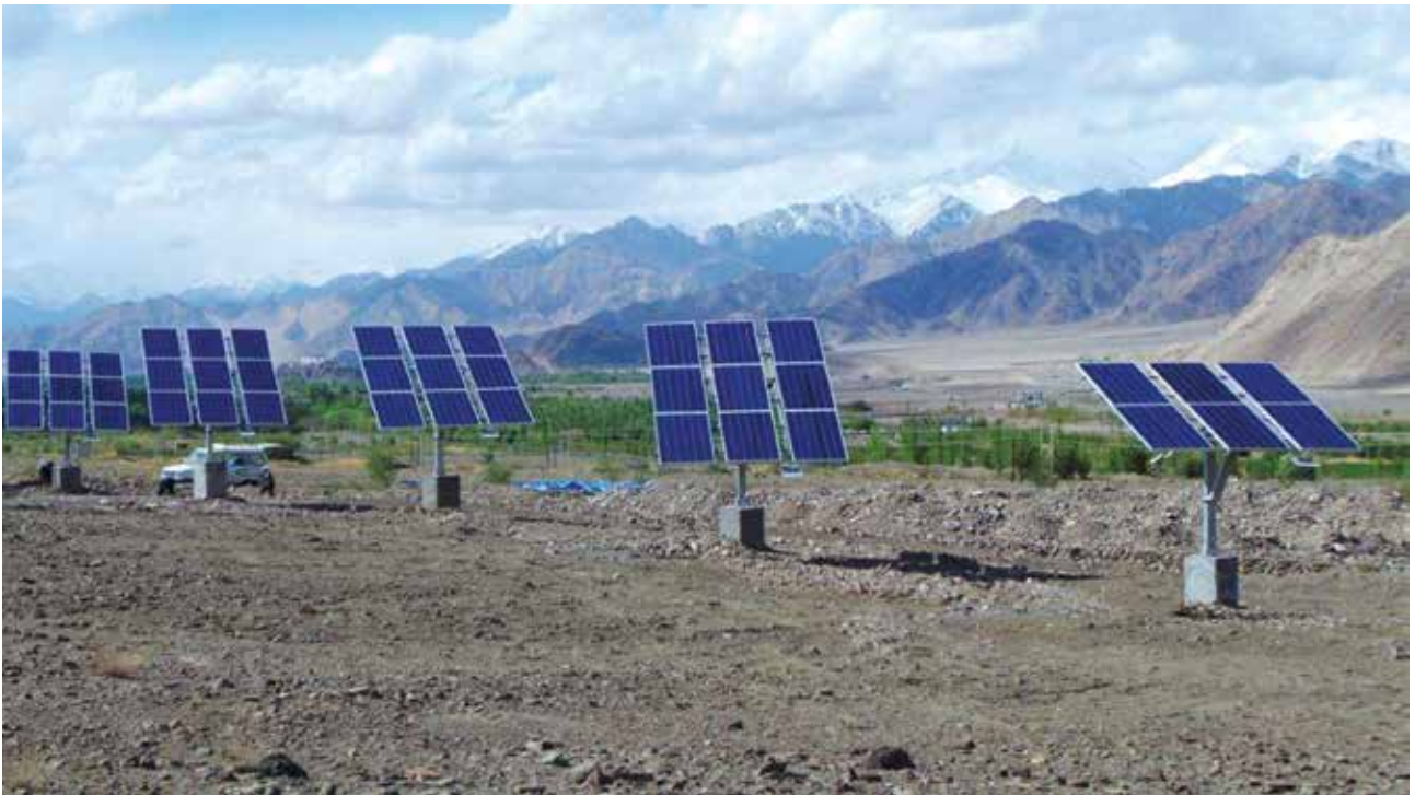
Solar powered pumps for sprinkler irrigation, installed at Leh, J&K. These pumps in the Himalayan Ranges are the highest such installations in the world.
